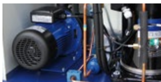
Pump P3 (3 barg) / P5 pump (5 barg, optional).
